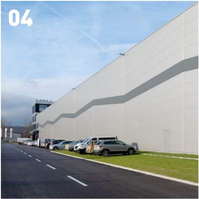
Diagonally installed Trimoterm FTV HL panels are up to 14m long.
